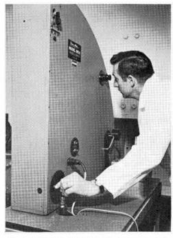
L. E. HEAMES (5134-1) is focusing and aligning framing camera for forthcoming shot. Thick laminated glass in small opening protects camera lens from shrapnel.
